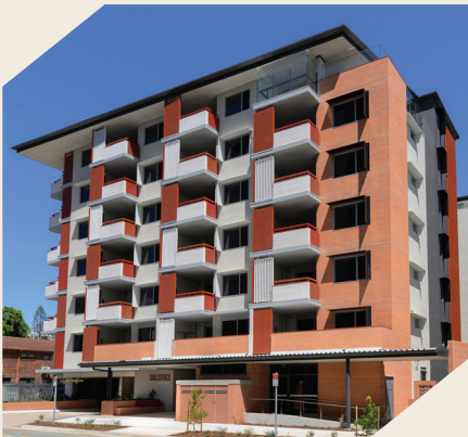
Redcliffe housing development, Brisbane, Qld.
